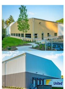
Hance Construction coordinated design, fabrication and erection of this 74,000 SF warehouse with 8,000 SF of office space in Hawthorne, New York. The building is a 216' wide space with minimal interior columns (2 rows), utilizing 50' Butler Landmark 2000 truss purlins.
