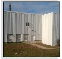
All of the new trims were custom field bent and cut out of flat-stock material with the exception of standard J-trim and base trim that was used over the doors, windows, louvers, and at the base of the walls.
