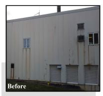
The East Brunswick Director of Public Works wanted their existing building retrofitted with new exterior paneling. They chose to have Butler Shadowall™ installed over a new 3" layer of insulation.
